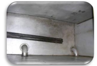
Tank Interior After Varnish Mitigation Service
