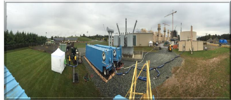
Staging Area Overview for Phase 1
