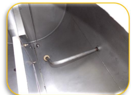
Reservoir After Chemical Cleaning
