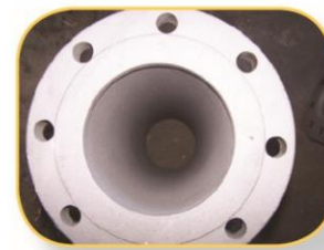
Chemically Cleaned 4" Line
