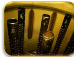
Filter Housing Before Varnish Mitigation Service
